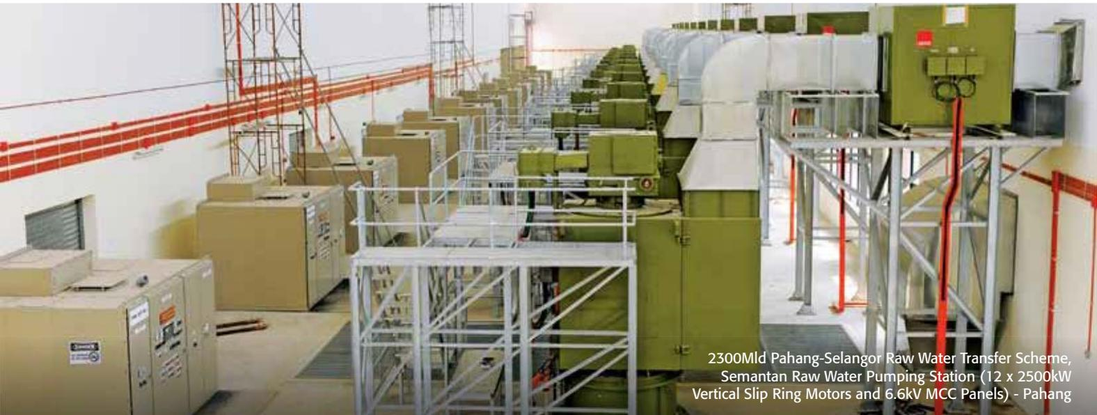
2300Mld Pahang-Selangor Raw Water Transfer Scheme, Semantan Raw Water Pumping Station (12 x 2500kW Vertical Slip Ring Motors and 6.6kV MCC Panels) - Pahang
