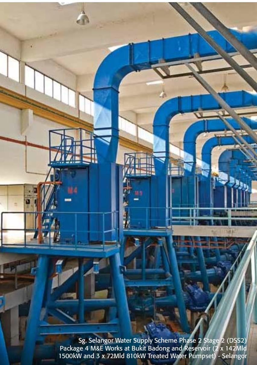
Sg. Selangor Water Supply Scheme Phase 2 Stage 2 (DSS2) Package 4 M&E Works at Bukit Badong and Reservoir (2 x 142Mld 1500kW and 3 x 72Mld 810kW Treated Water Pumpset) - Selangor
