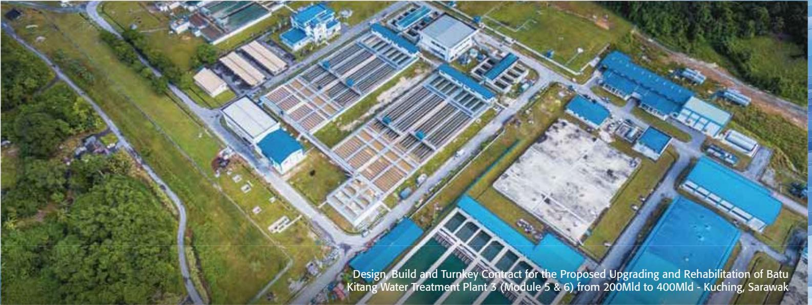
Design, Build and Turnkey Contract for the Proposed Upgrading and Rehabilitation of Batu Kitang Water Treatment Plant 3 (Module 5 & 6) from 200Mld to 400Mld - Kuching, Sarawak
