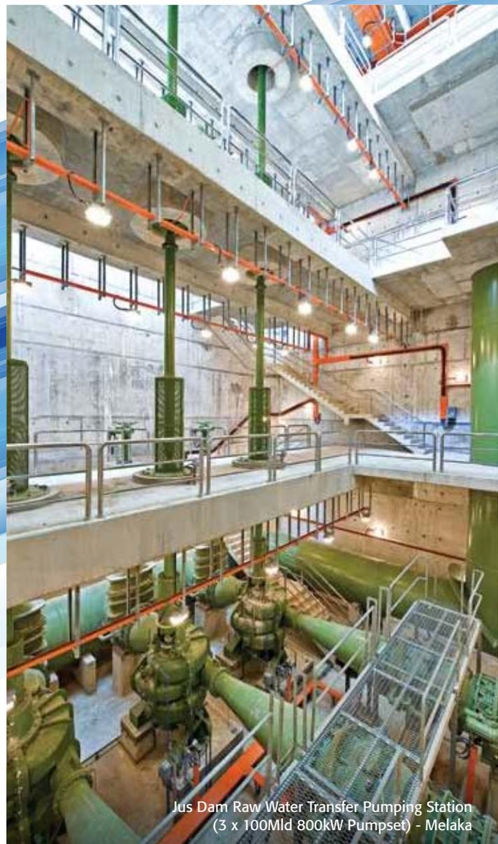
Jus Dam Raw Water Transfer Pumping Station (3 x 100Mld 800kW Pumpset) - Melaka
