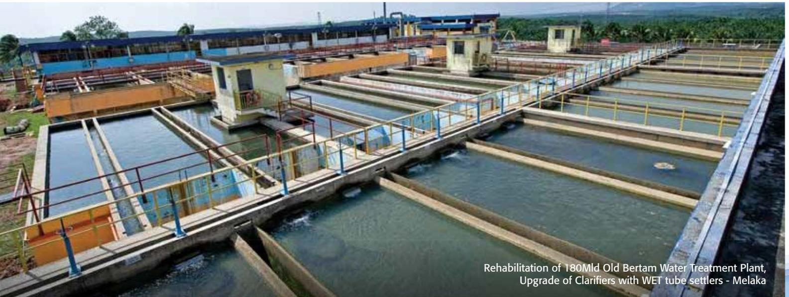
Rehabilitation of 180Mld Old Bertam Water Treatment Plant, Upgrade of Clarifiers with WET tube settlers - Melaka
